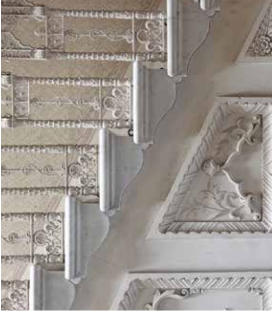
Detail of staircase, Elveden Estate, Suffolk.
